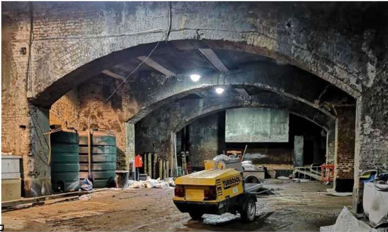
Removal of existing brick infill, smoke vent above retained
