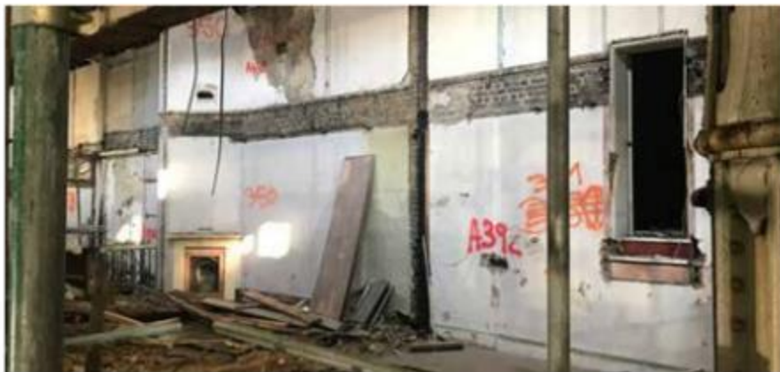
Existing spine wall condition
